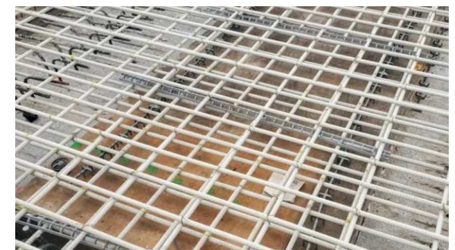
GFRP reinforcement for Harker's Island Bridge
