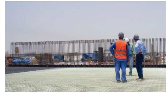
Floor slab, Qatar
