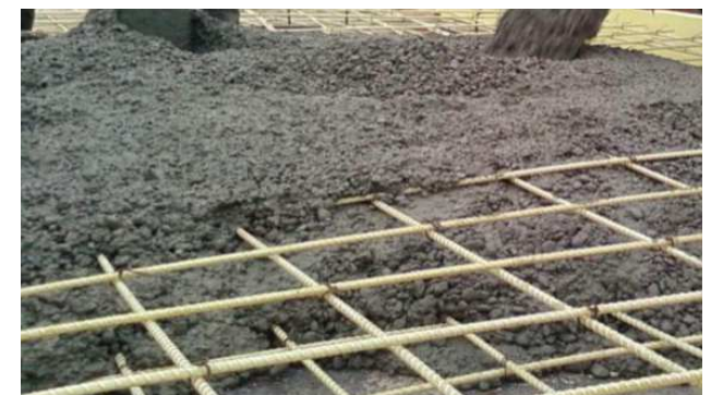
Base slab, private house
