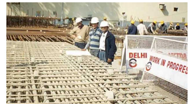
Subway project, India
