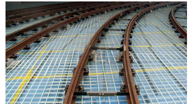
Floor slab railway depot Basel, Switzerland
