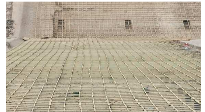
Jizan Flood Mitigation Channel
